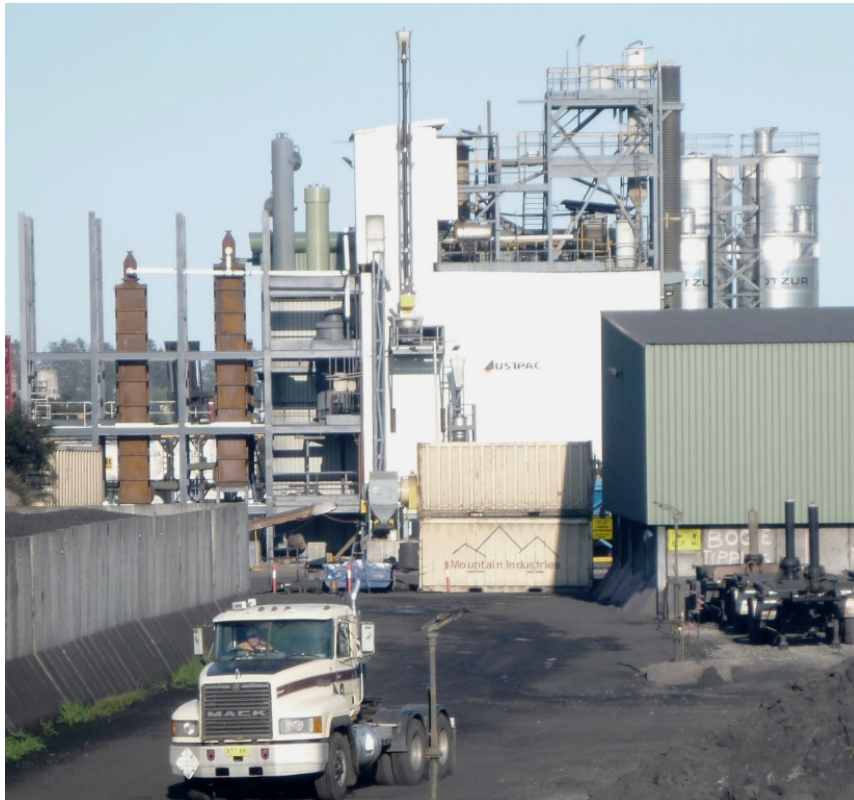
A view of the Newcastle Iron Recovery Plant (NIRP) from the west.
