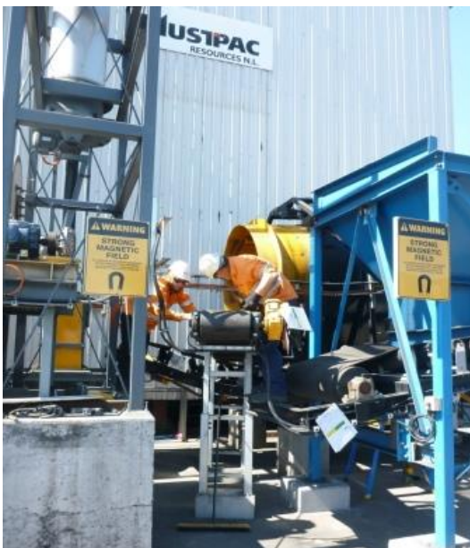
Adjusting conveyor belt tension prior to commissioning.
