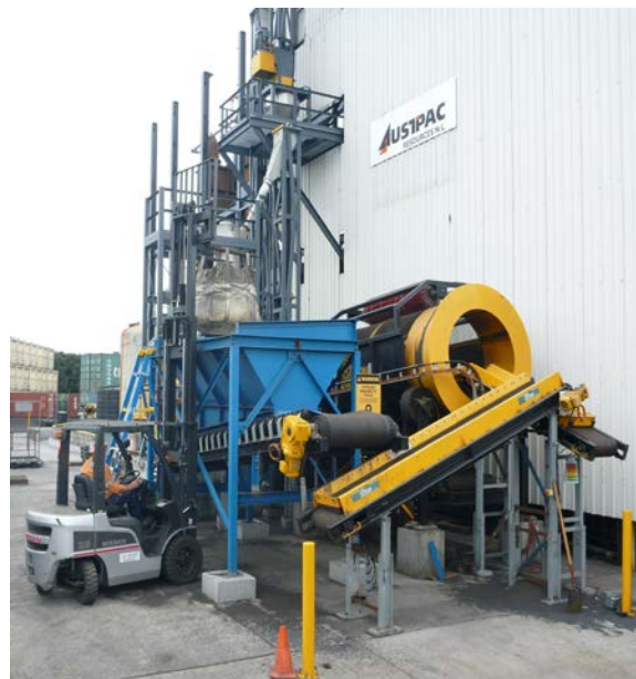
Charging the mill scale hopper.
