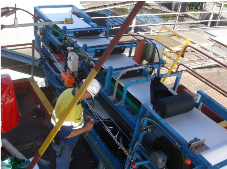
Delkor engineer installing and commissioning the Vacuum Belt Filter
