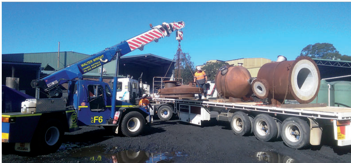
Unloading the caps and plenums (bases) for the two roasters
