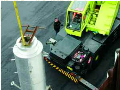
Installation of ERMS afterburner
