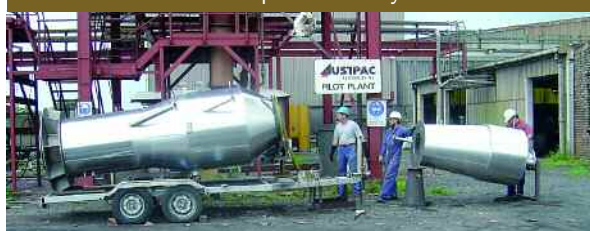
Oxidation roaster and pre-heater ready for installation
