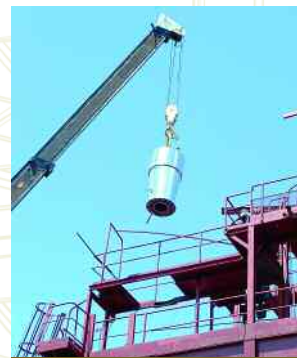
Installation of pre-heater
