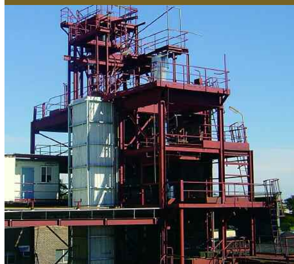
Construction of materials hoist shaft
